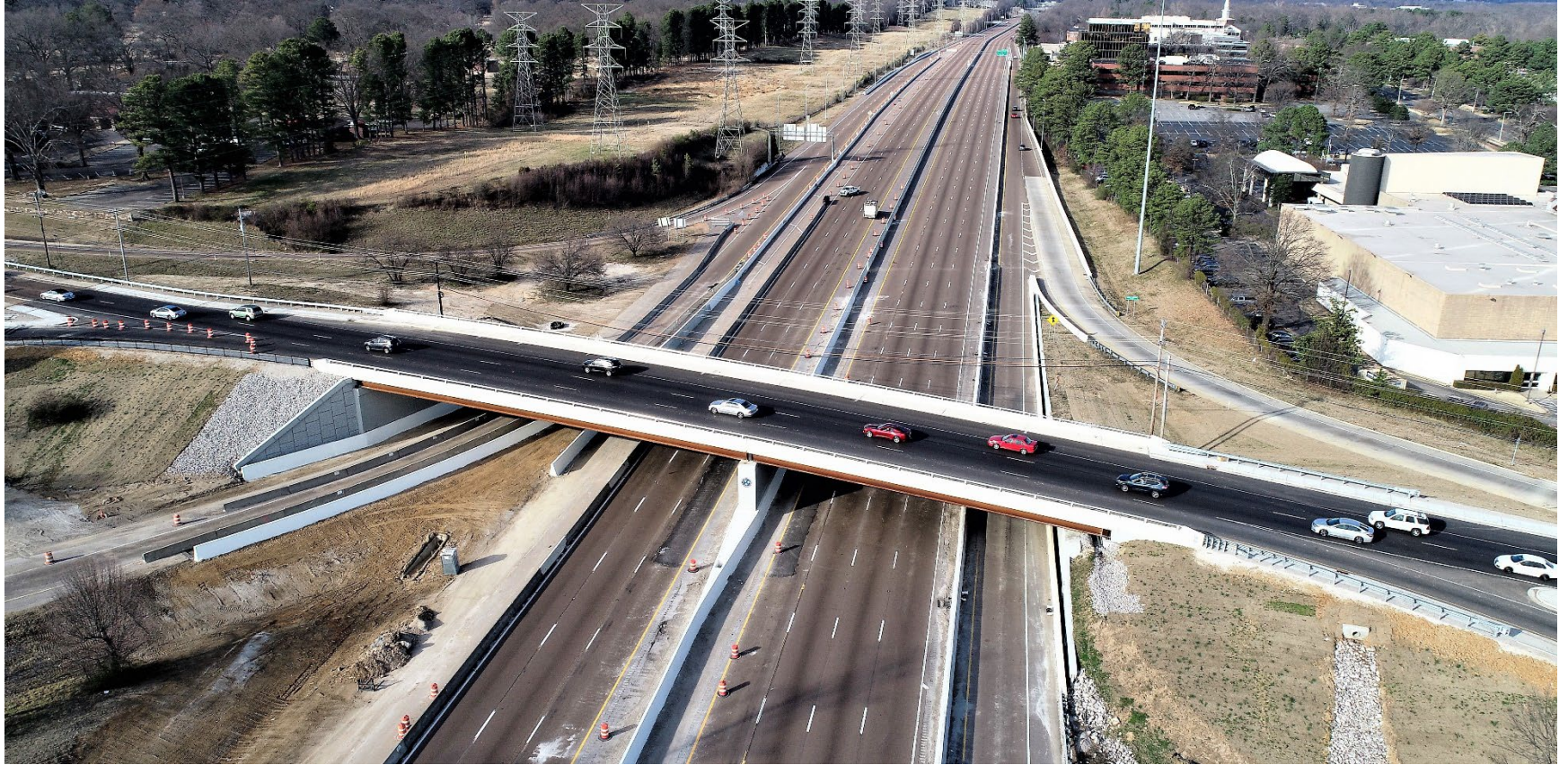
263' – 2 Span Steel Girder Bridge
